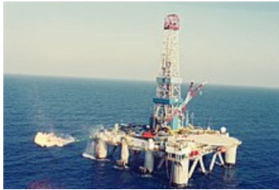
Noa natural gas field, offshore Ashkelon
